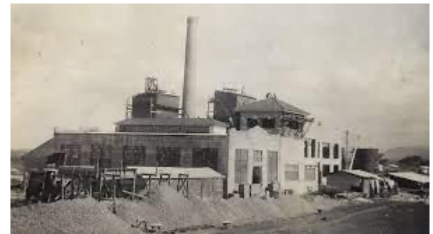
Powerhouse at Kahuku
